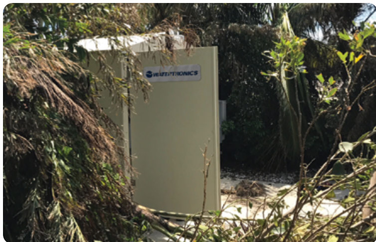
This composite enclosure in Naples, FL, withstood the impact of Hurricane Irma in 2017.
